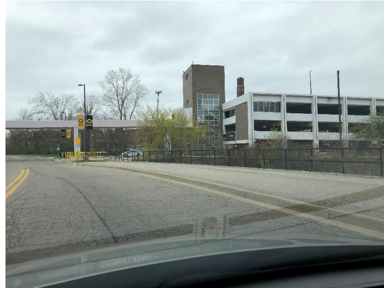
Parking Structures (G)
